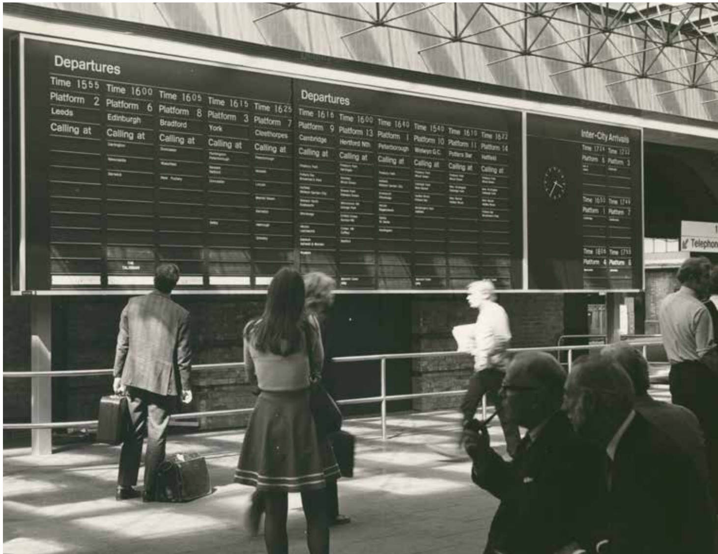
From 1954 Gino Valle, working also with John Myer, created clocks for Italian organisation Solari using the electro-mechanical 'flip' system. The classic form of this timepiece is the Cifra 3 . Britain's railways installed Solari devices in stations constructed or rebuilt in the 1960s and 1970s, including London Euston ( opposite ), Birmingham New Street, and London Kings Cross ( above ).
