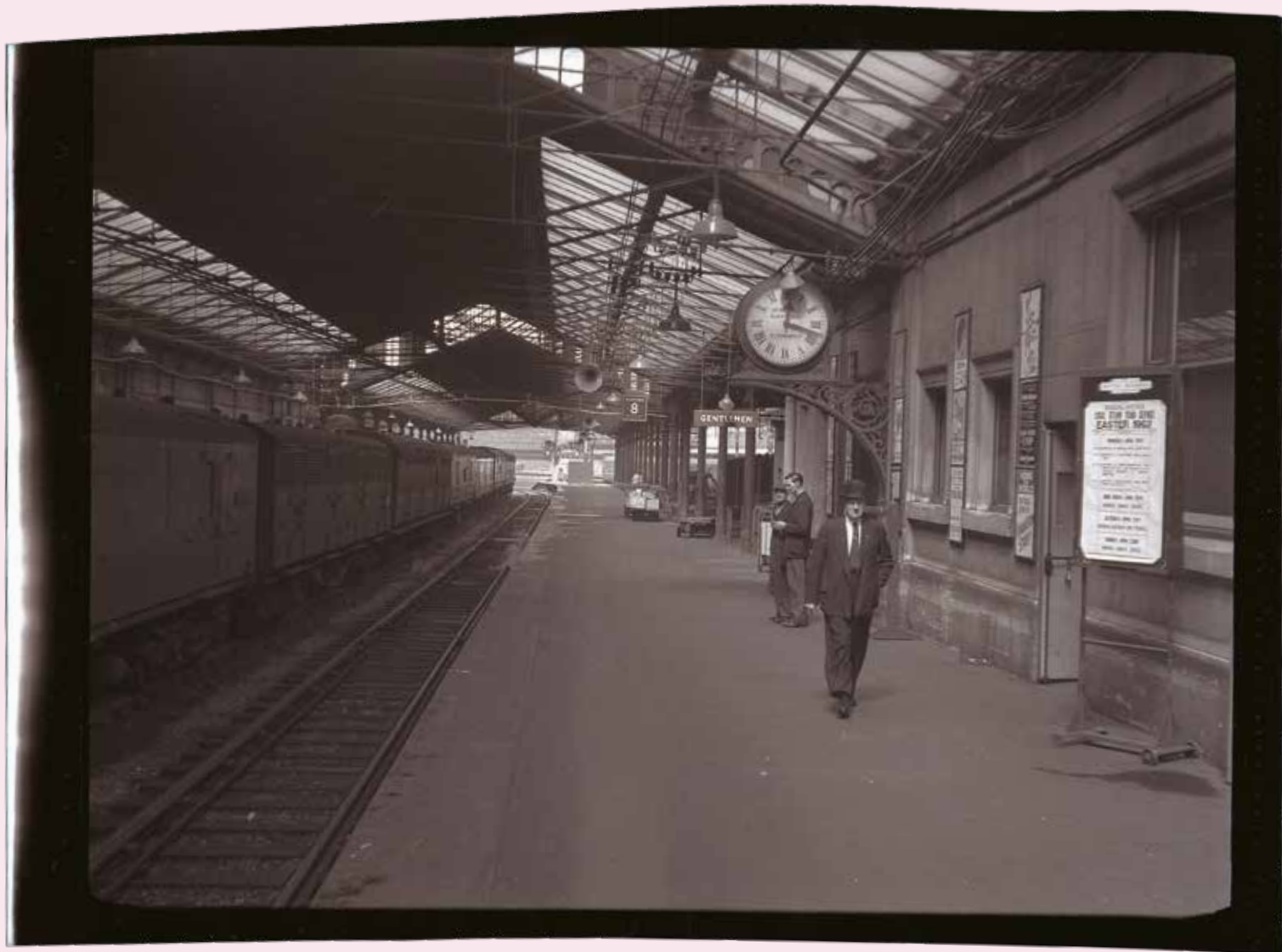
If a clock was in a location where it could not easily be seen from a distance, it could project at right angles from the façade on metal brackets laced together with arabesques and scrolls. This is the old Euston Station, London, 1962.
