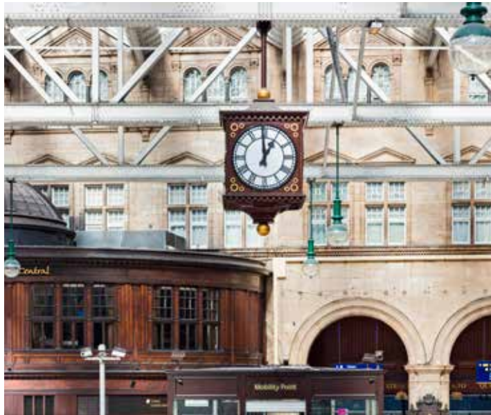
Glasgow Central, Scotland, rebuilt 1901–5.
