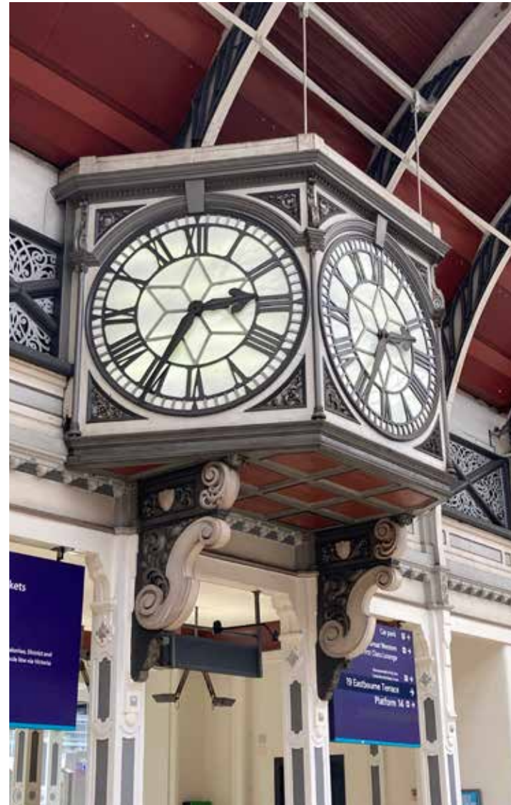
Paddington, over the loggia or 'Clock Arch' forming the original main entrance to the station. Installed around 1854 and restored 1985, this was the largest triple-dial clock in Britain.
